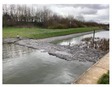
It is however clear that this section is still leaking, with water levels noticeably lower than other sections.
